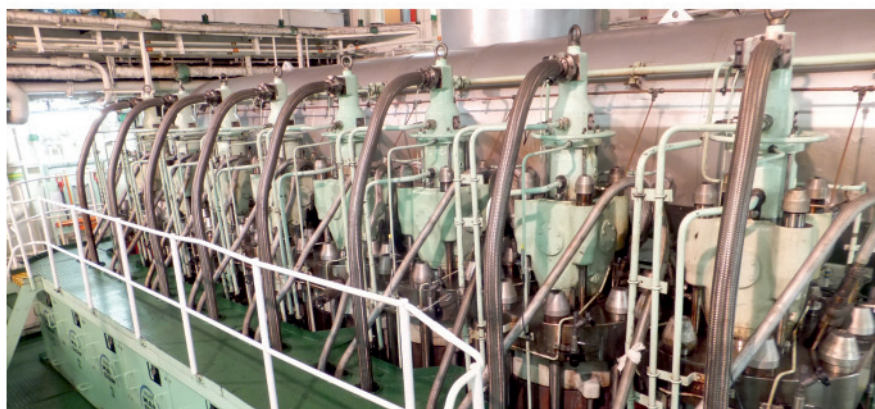
Fixed installed TCS-01CA sensors on a MAN B&W 2-stroke engine
